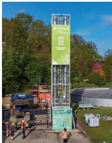
Carbon capture pilot plant
